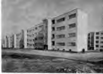
STEVEN BRONSTEIN: HOUSES FOR THE MODERN MAN, CHICAGO, 1945 The long bands of windows are made possible by steel construction. The most interesting part of the total program of the apartment block is regularity, consistency, orderliness. The repetition of the window line, or the other hand, gives an interesting variety to the general scheme of regularity.
