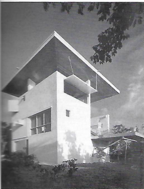
7. Frank Harmon and Associates, Taylor House Scotland Cay, Bahamas. The inverted roof captures the rainwater while shutters and sliding doors provide shade and protection from hurricanes (2001). (Photo by James West.)
