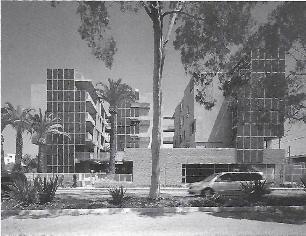
9. Pugh and Scarpa, Colorado Court, Santa Monica, California. View into courtyard framed by photovoltaic panels (2001). (Photo Courtesy of Pugh and Scarpa)
