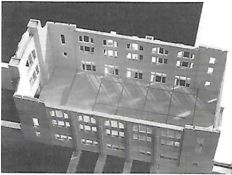
2. Model of building shell after demolition.
